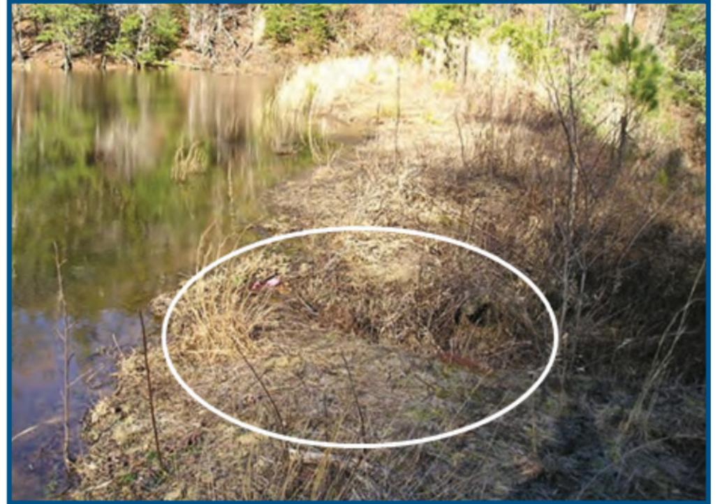
Figure 44 – Low areas in the crest of a dam reduce the freeboard (therefore allowing overtopping at a lower frequency flood).
