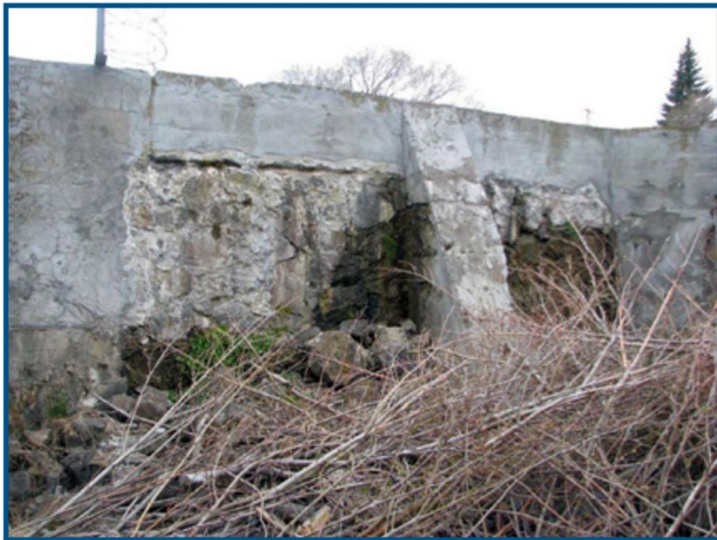
Figure 51 – Concrete deterioration on the downstream face of a dam.
