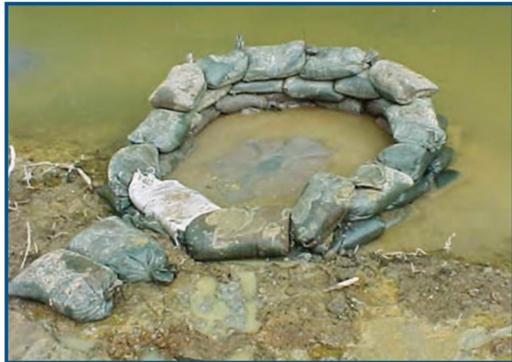
Figure 22 – Sandbags surrounding a boil on the downstream side of the dam (note the mound of material forming in the center of the sand-bagged area).
