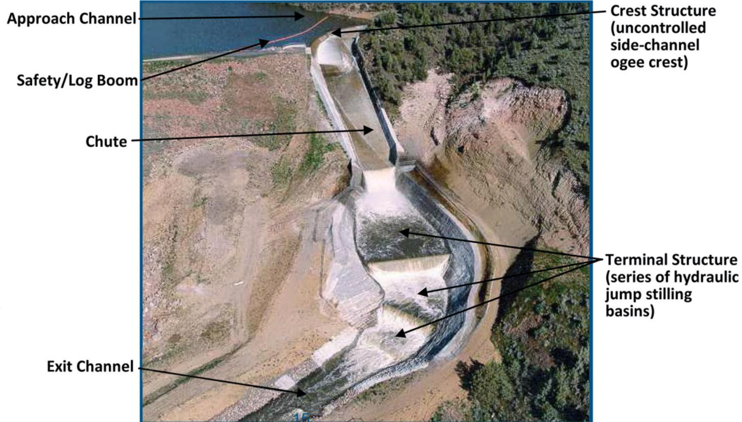
Figure 16 – Spillway Overview with structures identified.
