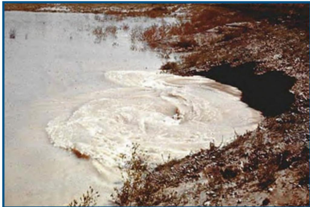
Figure 26 – Whirlpool action in the reservoir (unrelated to an outlet works intake) could be an indication of advanced piping. Dam failure could be imminent.
