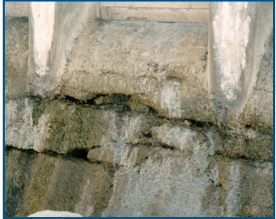
Figure 50 – Open joints.
