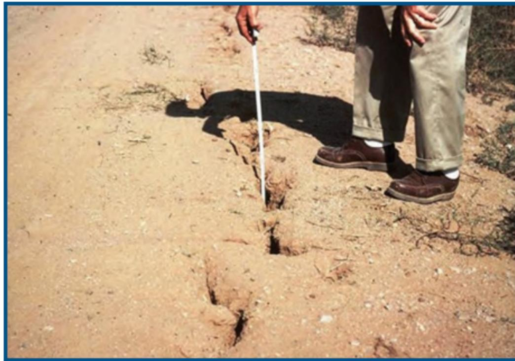
Figure 32 – Longitudinal cracks can be an indication of dam instability.
