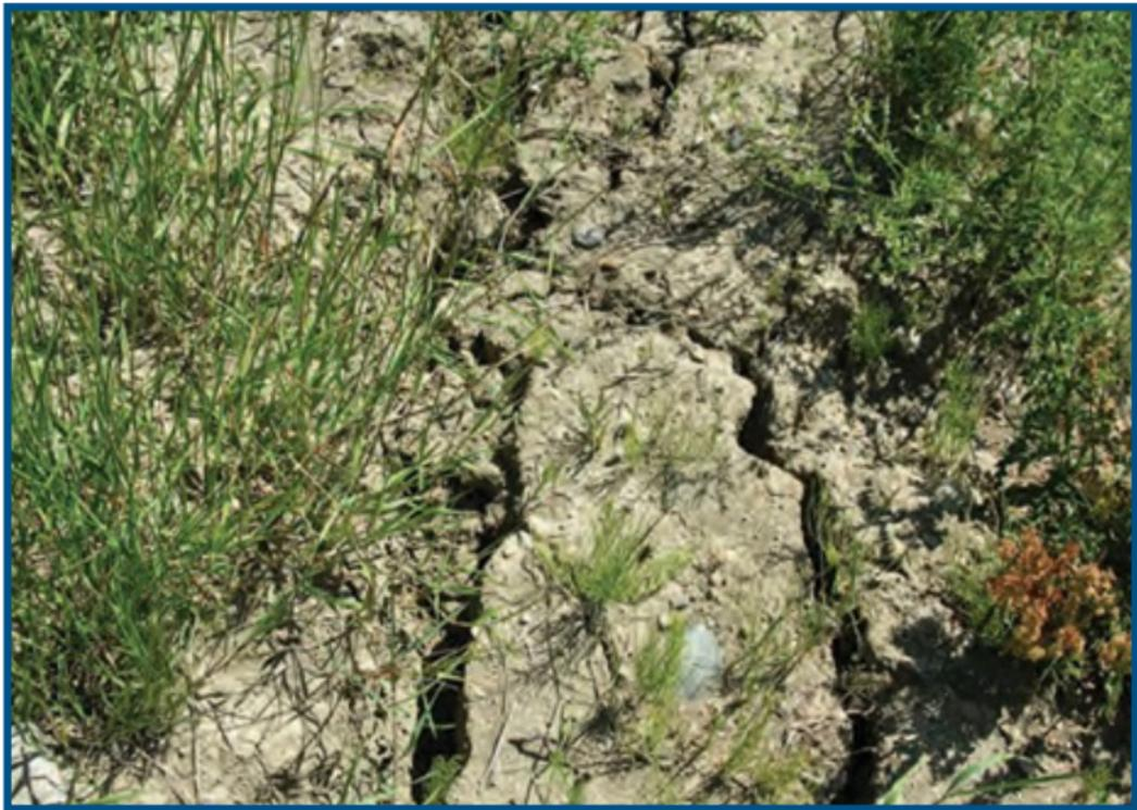
Figure 30 – Transverse cracks may provide open seepage paths through an embankment dam.
