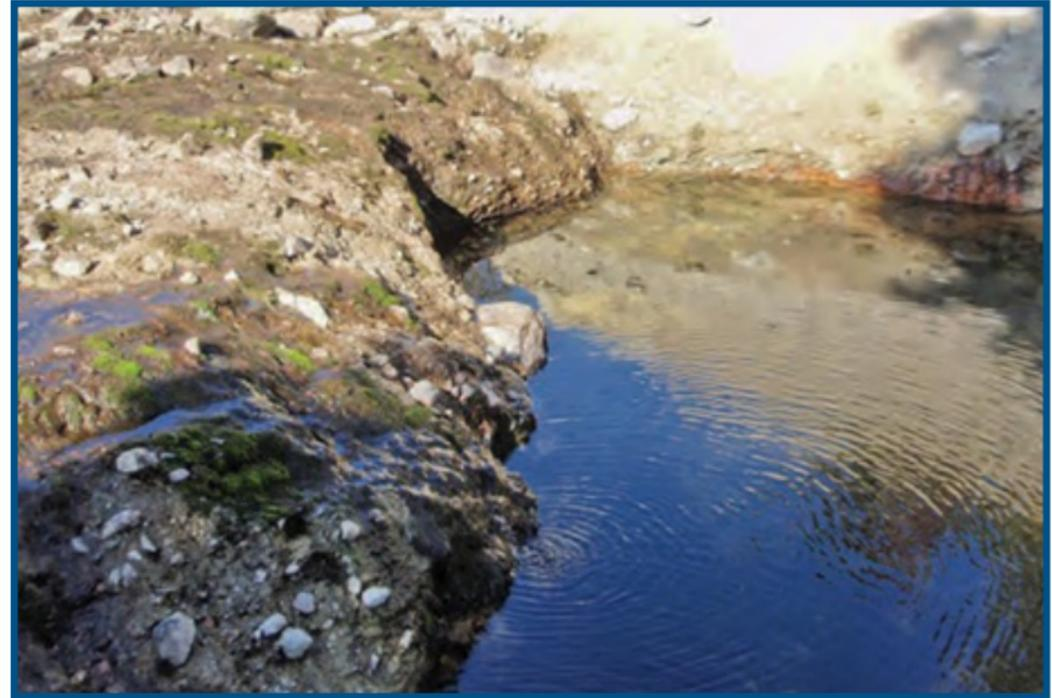
Figure 56 – Erosion of the spillway channel may lead to slumps or slides of the spillway sides, or large, uncontrolled, unintended releases in the event erosional headcutting in the spillway channel breaches the spillway crest.
