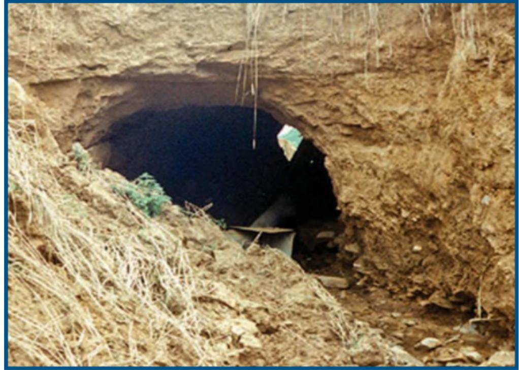
Figure 20 – Embankment erosion adjacent to an outlet pipe.
