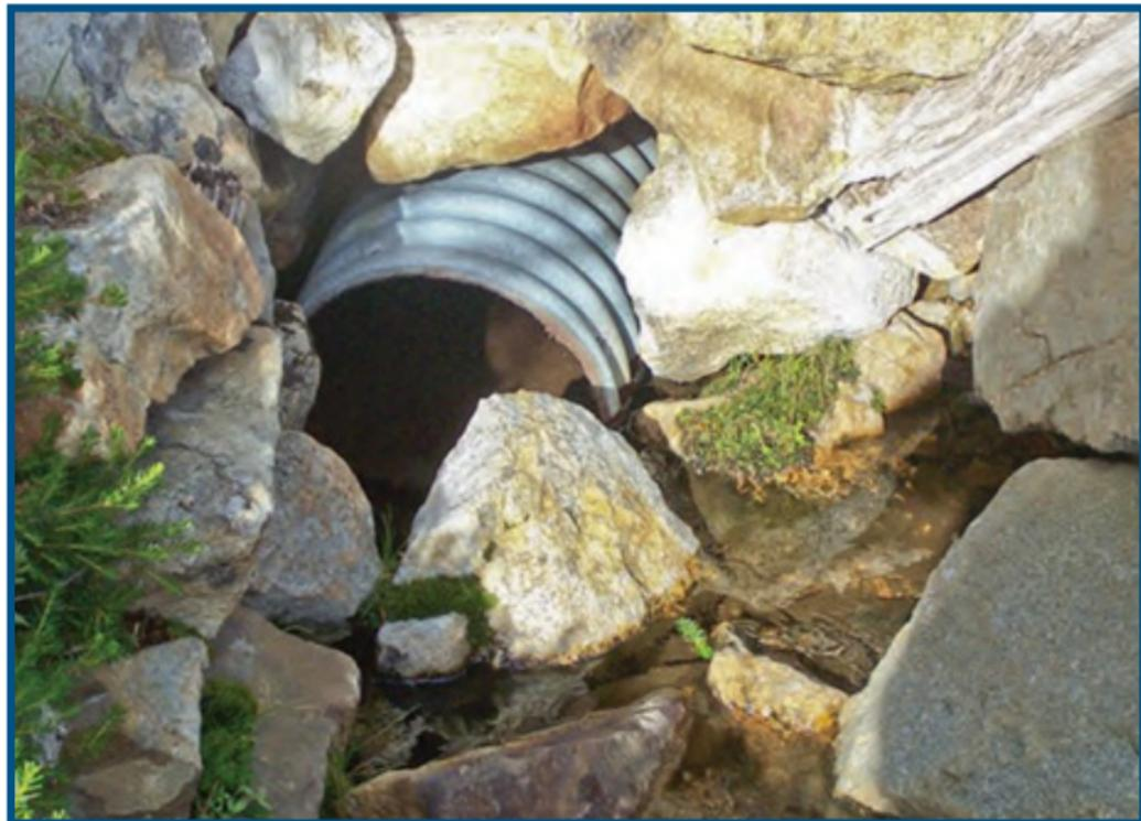
Figure 46 – Rock blocking discharge of an outlet
