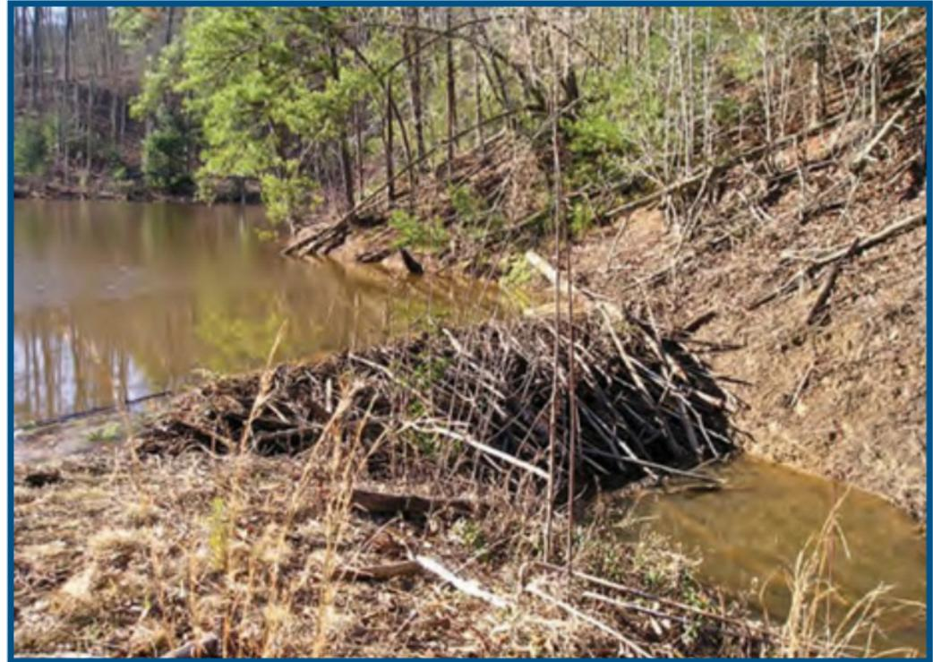
Figure 54 – A blocked spillway channel may cause overtopping of the dam due to the loss of the spillway discharge capability.
