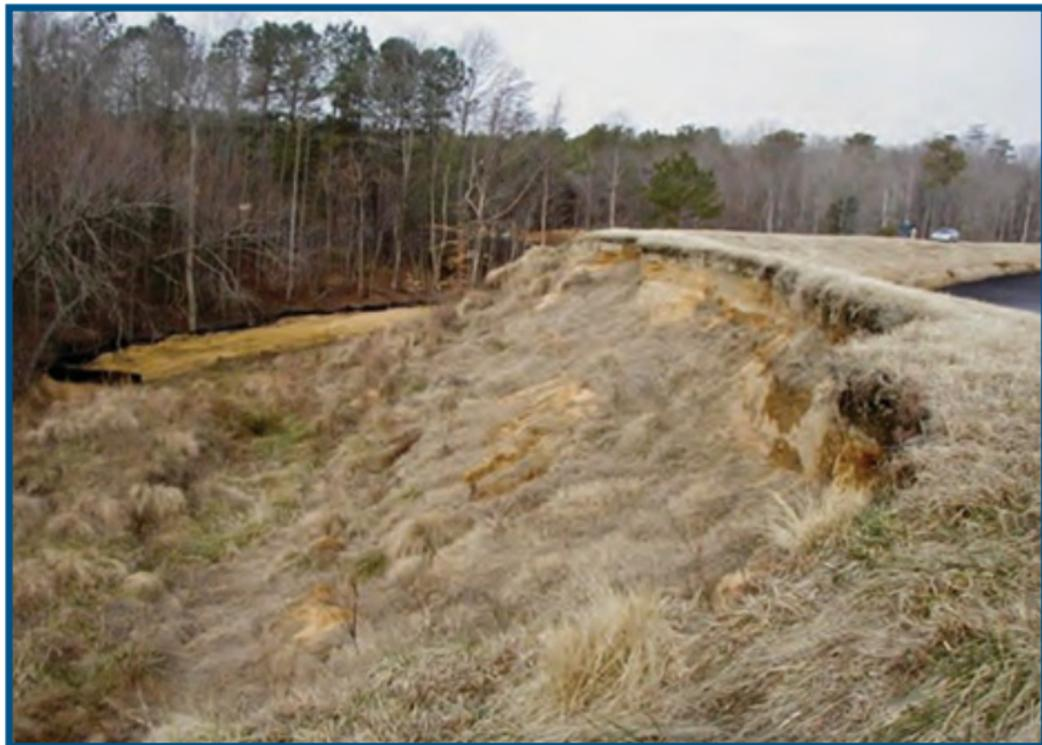
Figure 28 – Slumping on the downstream face of a dam.
